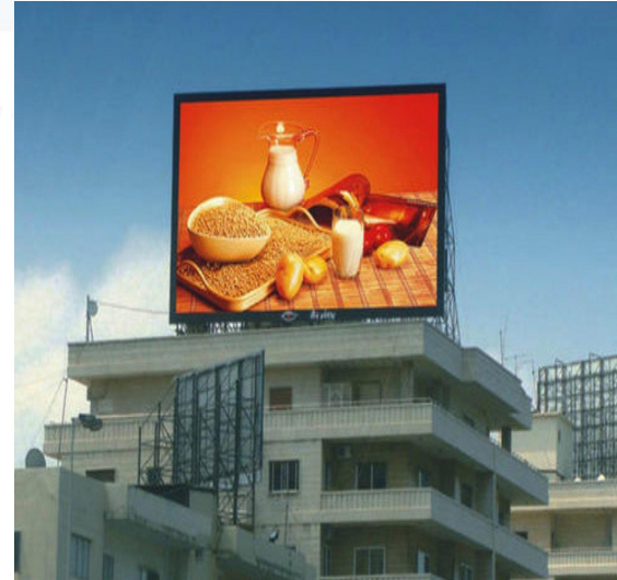
Back Support Installation
